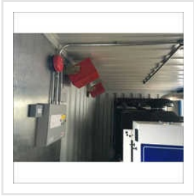
Aerosol Based Fire Suppression System
