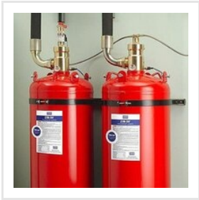
Fk 5112 Fire Suppression System
