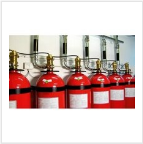
Hfc 227ea Auto Fire Extinguishing System
